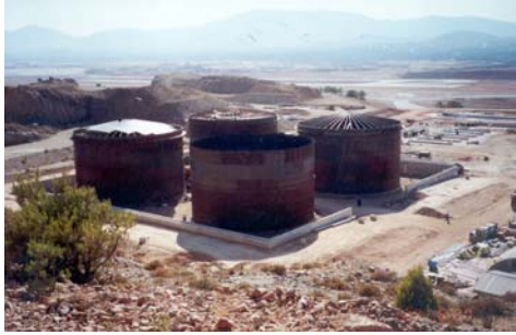
4x6.000 m 3 Fuel Storage Tanks ATHENS INTERNATIONAL AIRPORT
