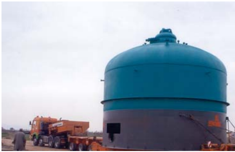
F.E.A. of a Top FCC Reactor for Refractory Lining Integrity During Transportation and Erection (HELPE)
