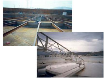
80.000 m 3 Fuel Storage Tank during construction (HELPE)
